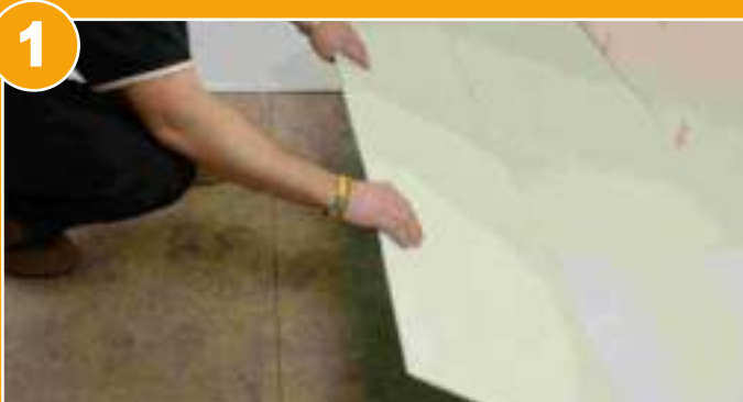
After preparing a smooth surface, measure the area to be heated. Fit the ECOMAX-LITE Insulated Tile Backer Board (available separately) to the floor securely following the manufacturers instructions.
