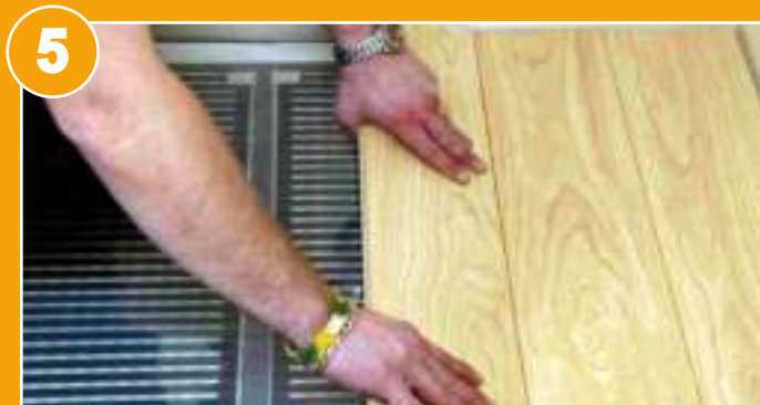
Lay the floor covering as soon as possible to prevent damage to the element.
