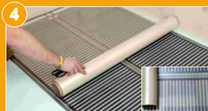
Cover the total ECO FILM SET installation with POLYESTER VAPOUR BARRIER (available separately).
